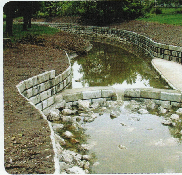
Construction workers installed approximately 38,000 sq ft of retaining walls on site.
